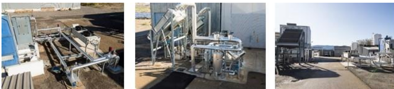
Figure 80. The PSA Cooling Facility. (lef) Wet Cooling tower and Air Cooled Heat Exchanger (Innovative Combined Cooling System); (centre) Steam generator connected to the Air Cooled Condenser and to the Surface Condenser; (right) General view of the Cooling Facility
