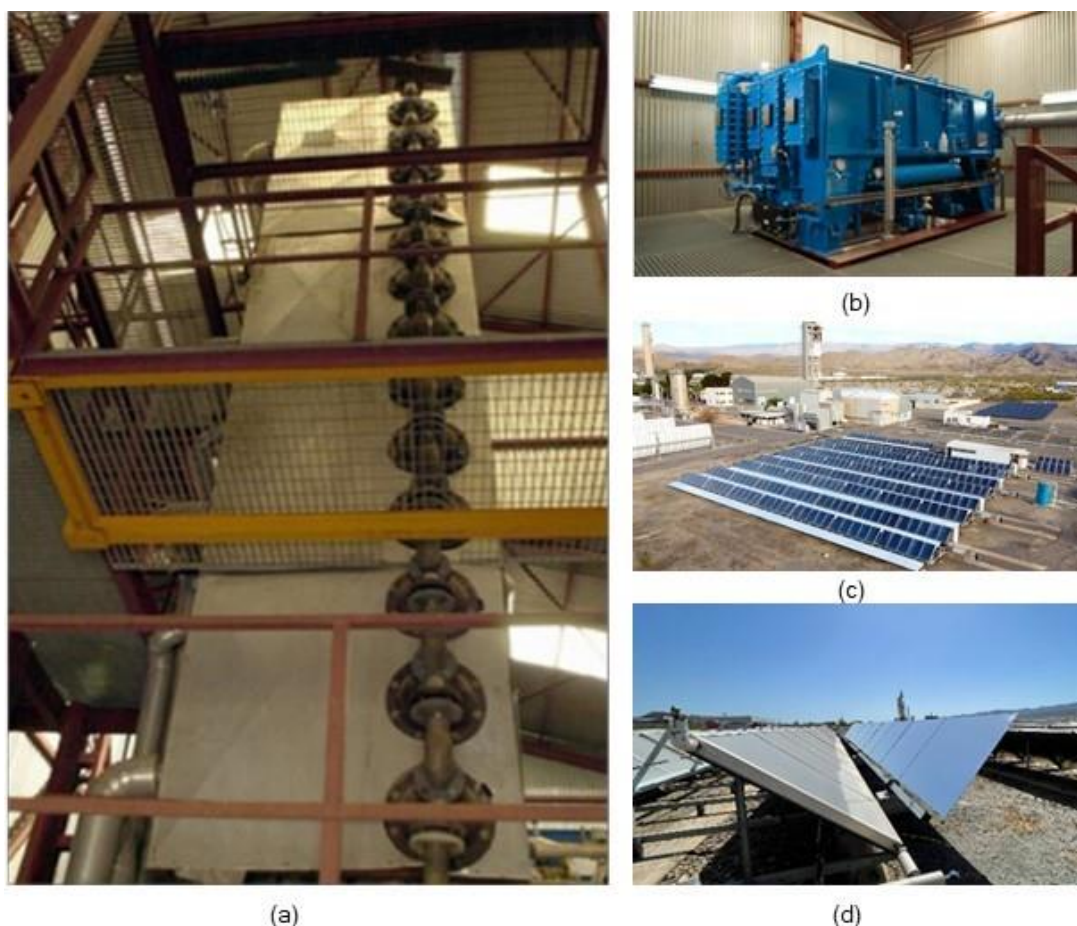
Figure 75. The PSA SOL-14 MED Plant (a) double-effect LiBr-H 2 O absorption heat pump (b) and 606-m 2 flat plate solar collector field with tracking mirrors (c and d).
